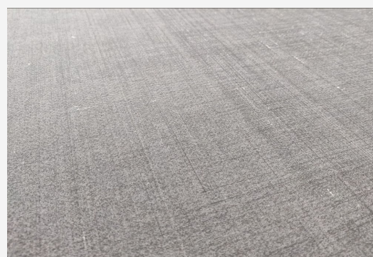
Example of proper cutting depth
